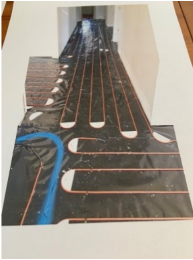
Figure 5. Typical floor heating installation.
